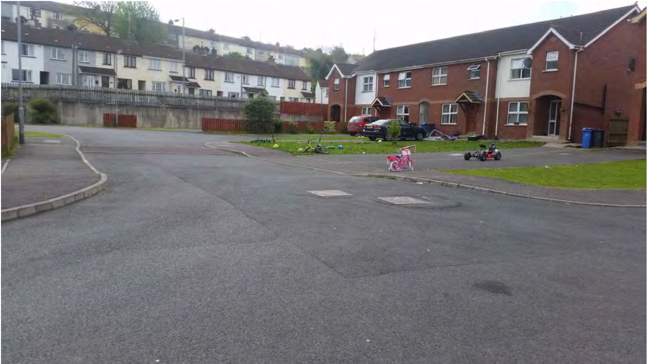
Plate 11 Road Surface at Manhole F4 and S3
