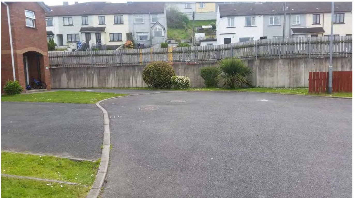
Plate 14 View of manholes S5/F5, with manhole reflecting through road surface
