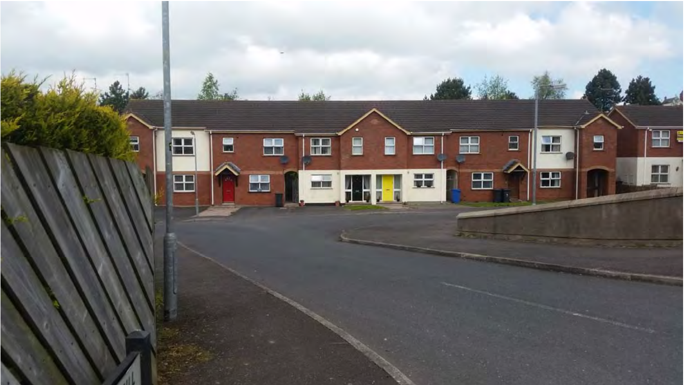
Plate 1 View of Site from Stream Street (House Nrs 6 to 11)
