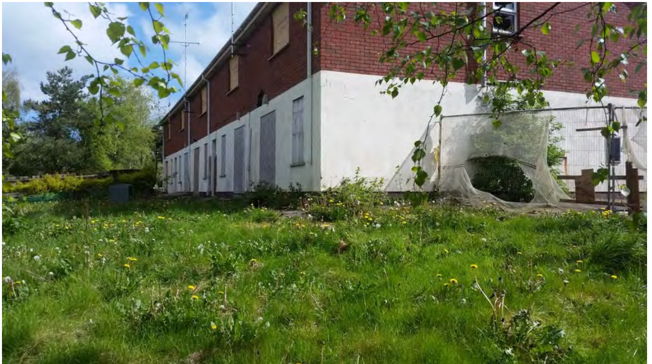
Plate 16 View of Rear to House Nrs 17 to 21
