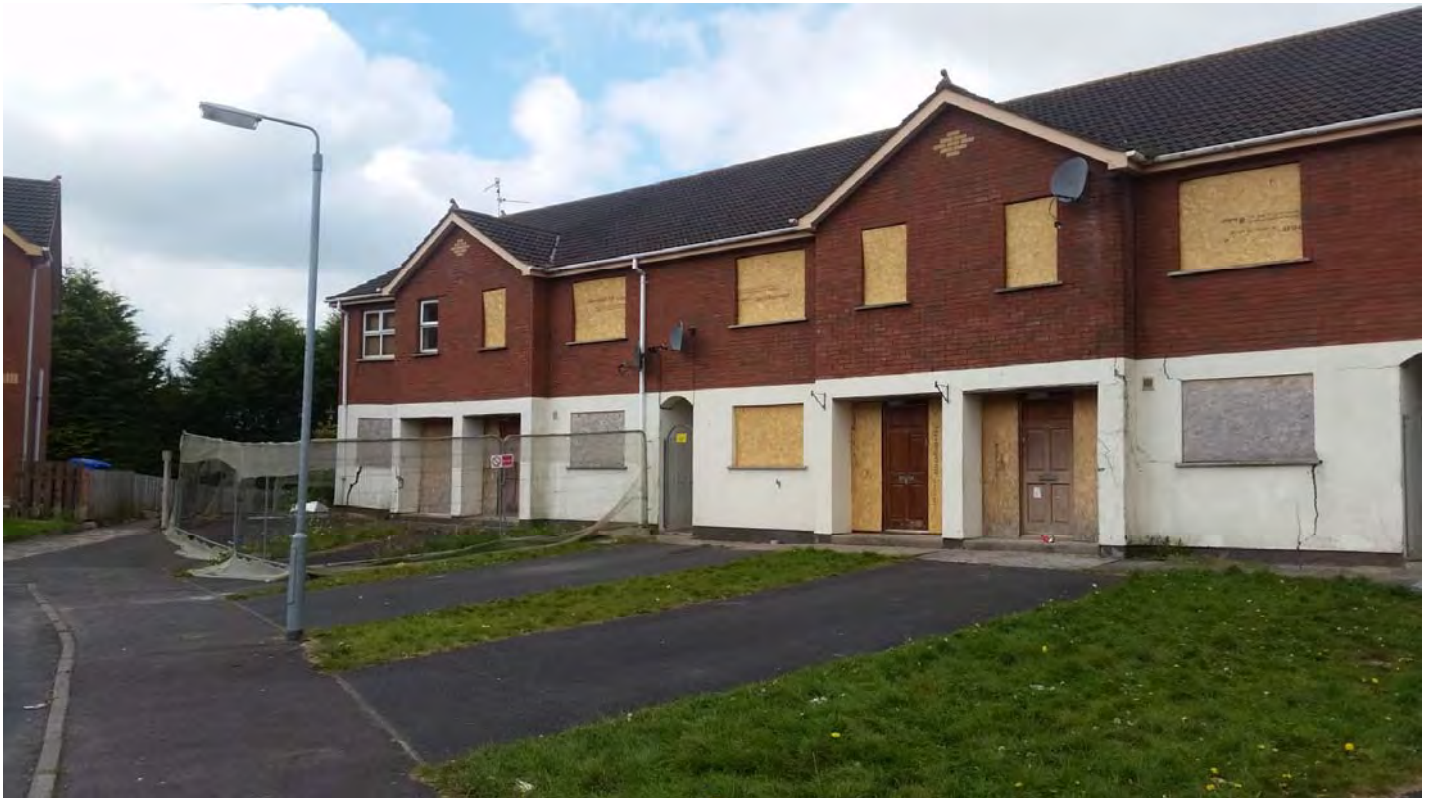
Plate 8 Severe Cracking House Nr's 17 to 21
